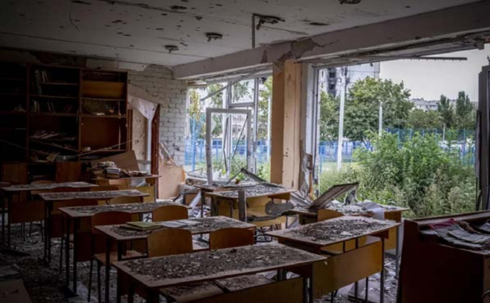
A damaged classroom in Saltivka, Kharkiv, an area badly affected by the war in Ukraine.
